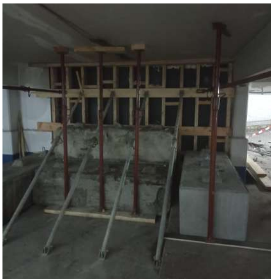
Figure 6: Comblement du tunnel A.
