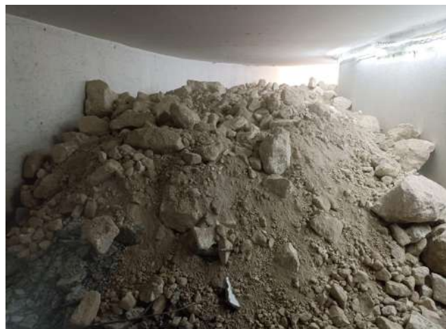
Figure 6: Comblement du tunnel A.
