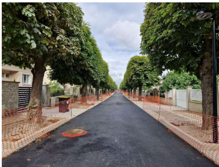
Figure 4 - Visite de chantier - Bvd Blanqui (A. Olivier, 2025)
