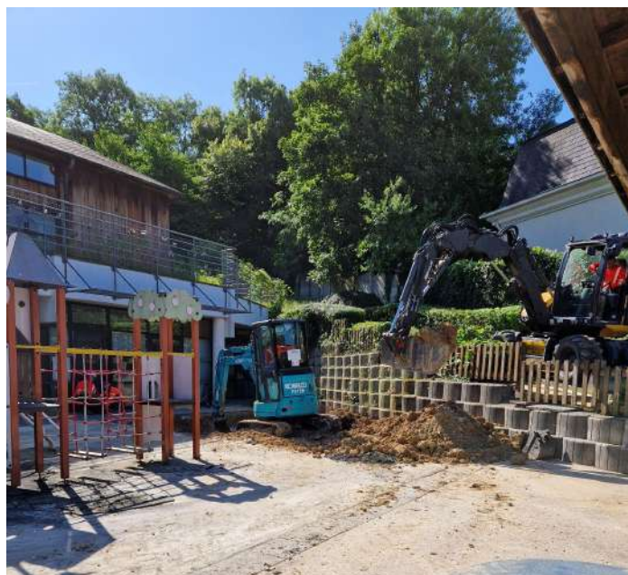
Figure 5 - Visite de chantier - École Daguerre (C. Guilmeau, 2025)
