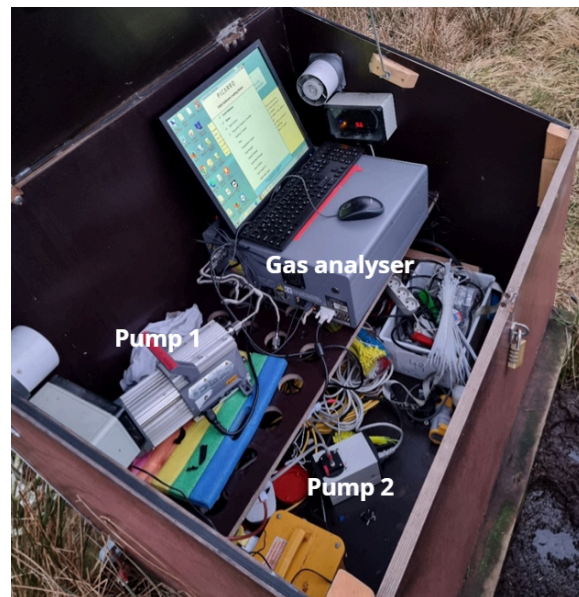
Figure 11 : Gas analyzer, Picarro model G2508 with circular airflow system driven by pumps. Pump 1 creates a constant vacuum inside the analyzer for correct pressure inside the analyzer. Pump 2, has a vacuum and pressure outlet, creating the airflow circulation in the system.
