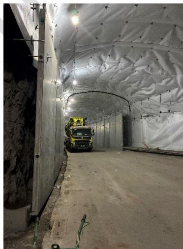
Figure 10: photo of the wall setting
