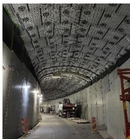
Before the shotcrete
