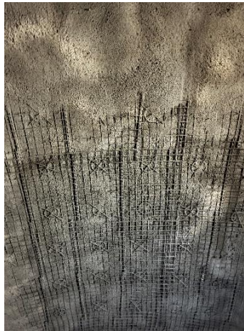
Figure 12: photo of a tunnel roof during the shotcrete (not finished)
