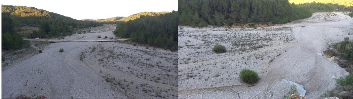
Figure 4: Photographs of the Rambla de la Viuda near the junction with the Carretera de Vilafamés a Costur.
