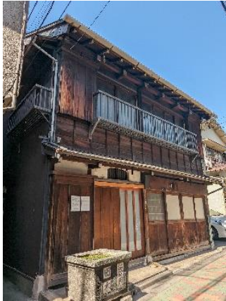
Figure 24: Former Iida house (Elsa MELEDO, 2024)
