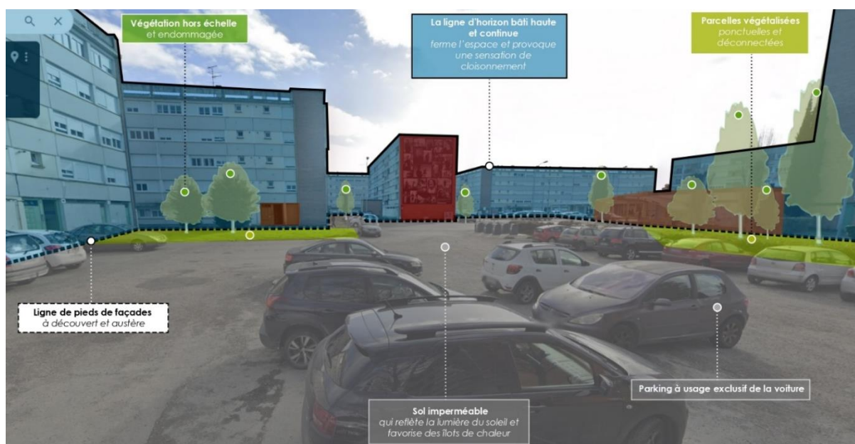
Figure 12: LAPANOUSE - Square Amiral Abrial - Existant
