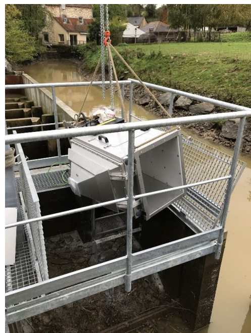
Figure 8 - Installation du Riverwatcher (@Syndicat JAVO)
