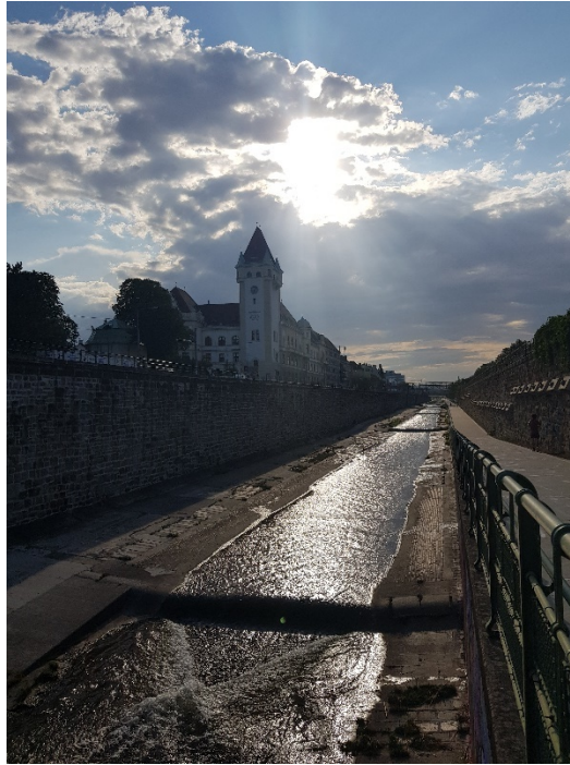
Figure 1: Artificial and heavily modified section of the Wien River with some of the migration barriers (concrete steps) at the Kennedybrücke station
