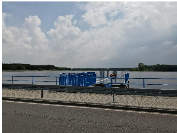
Figure 3: Photography of Smardzew Reservoir dam
