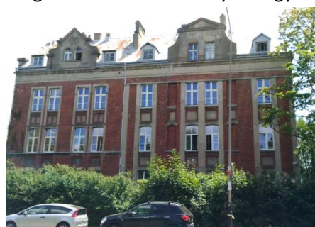
Figure 1 ERCE PAS building, source : Florian MIROLO
