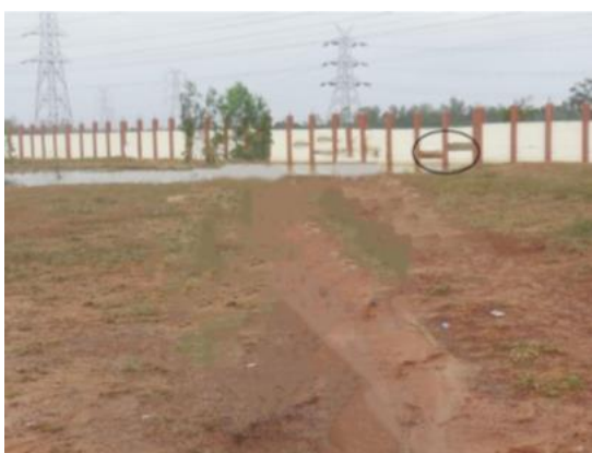
Figure 19 Panel in compound wall taken off to let water flow
