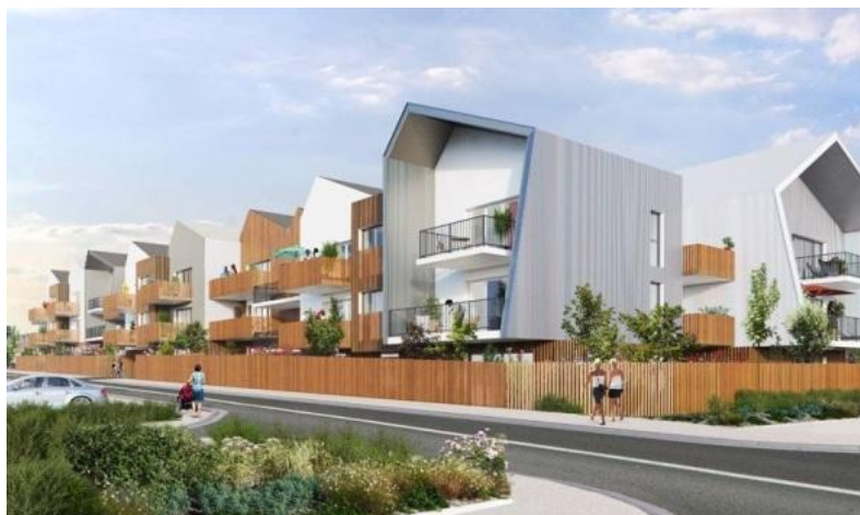
FIGURE 23: OPERATIONS IMMOBILIERES "LA GRAND'VOILE" ET "ONIA" DE BOUYGUES ET VINCI (SOURCES: BOUYGUES-IMMOBILIER.COM, 2017; VINCI-IMMOBILIER.COM, 2017)
