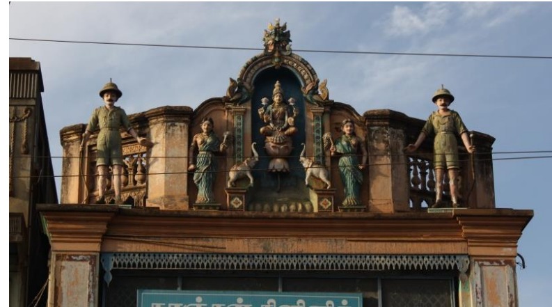
Figure 21 Details of a Karaikudi Chettiar facade with two British soldiers (photo by M.SINOUE)
