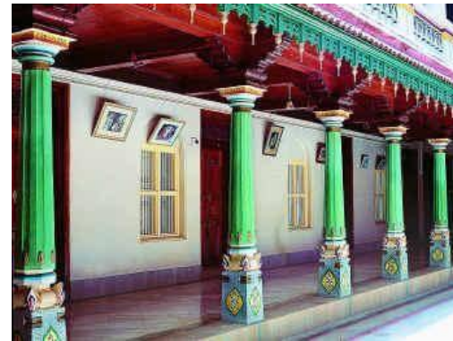
Figure 18 Pillars from the first courtyard in Chettinadu Mansion (photo by C.BUGEIA)
