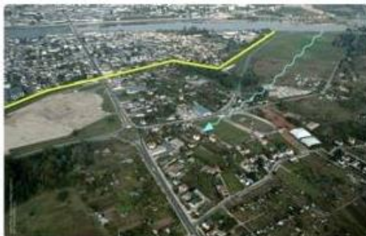
Figure 2. The built area located in the "Bouillie" discharge channel in 2006 (in the foreground).
