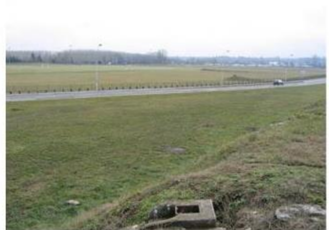
Figure 3. View of the discharge channel from the spillway Source : Mission Val de Loire (valdeloire.org)
