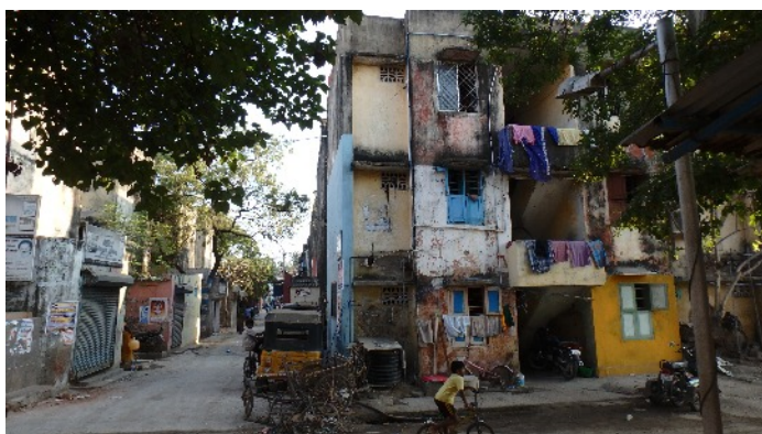
LIG BUILDING IN KOTTURPURAM SLUM CLEARANCE COLONY
