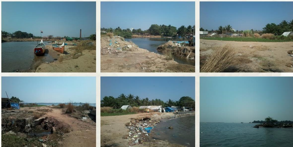
Fig 10: view of the stretch-1 of the mangalore corniche project, Source: Author (Field study)
