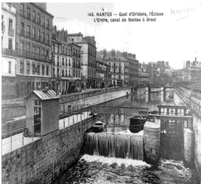
Fig 1.15: River L'Erdre in 1900 before the reclamation
