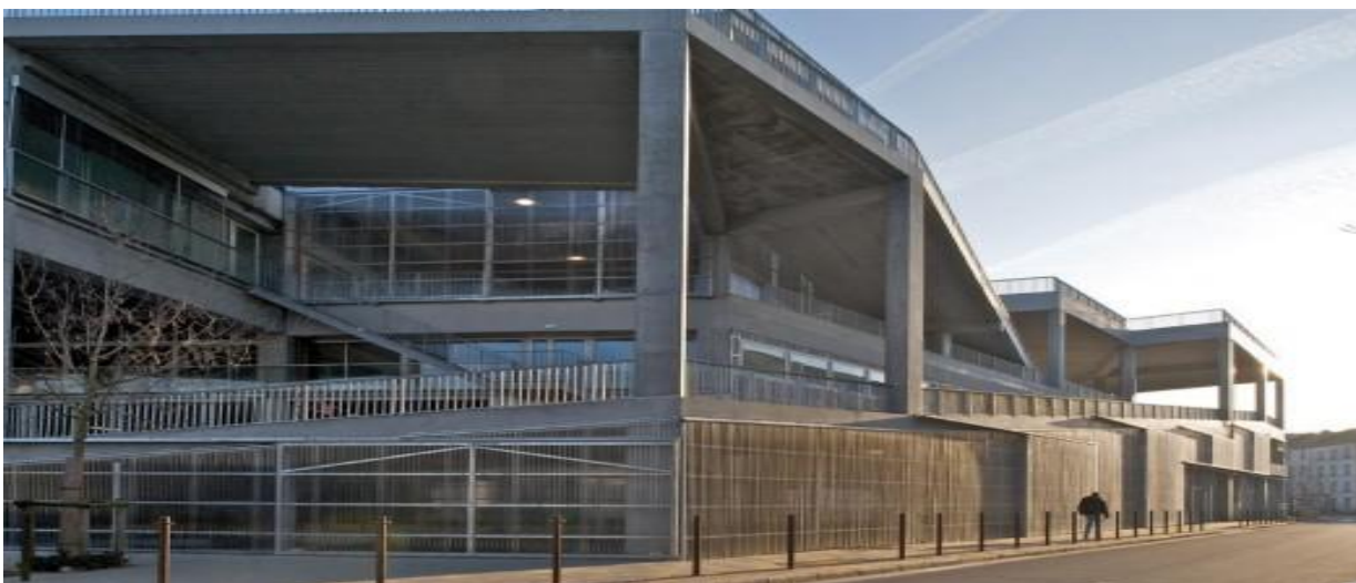
Fig 1.32: School of Architecture, Nantes
