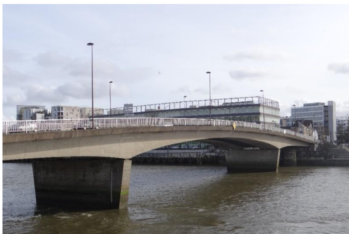
Fig 1.55: Bridge connecting the two banks
