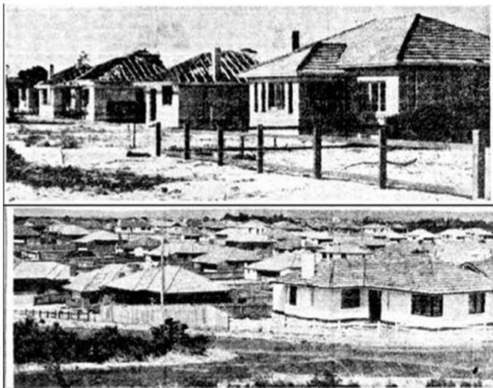
Figure 2, houses being built in Bayswater and South Perth from 1945-1948, source The west Australian 1952
