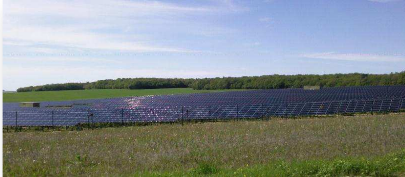
Image 8 : Champs photovoltaïques, Massangis
