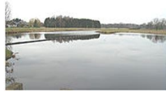
open retention basin
