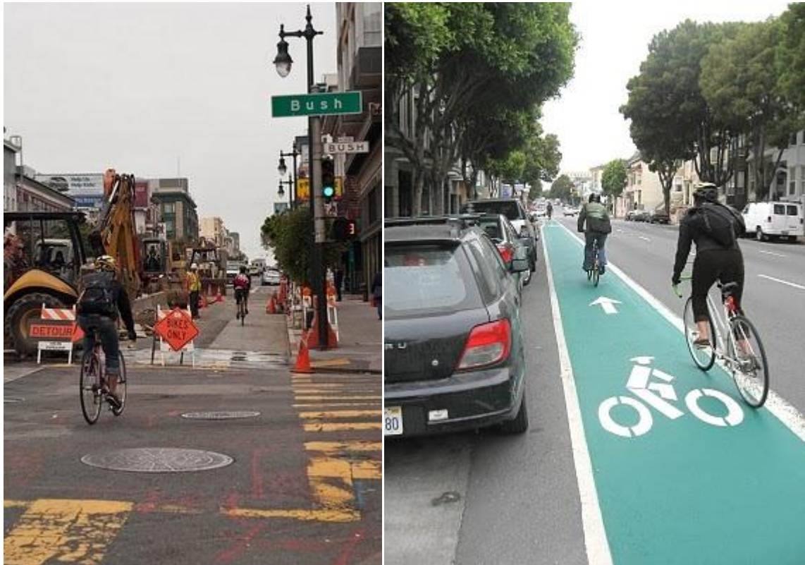
(Helquist, 2010) Bike Lane Construction and Completion on Valencia Street
