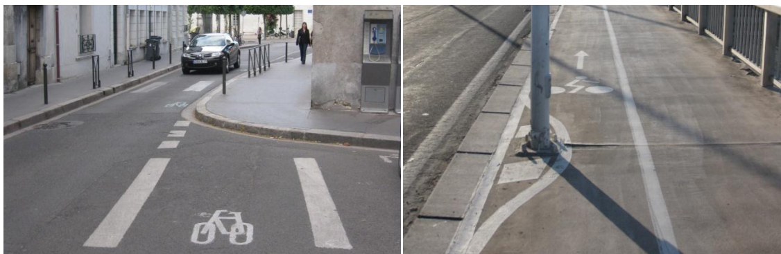
Rue Néricault Destouche Tours, France: Bike lane puts cyclist into a dangerous place. (Chapman) Puente de la Barqueta Seville, Spain: Light post in bike lane creating a safety hazard. (Chapman)
