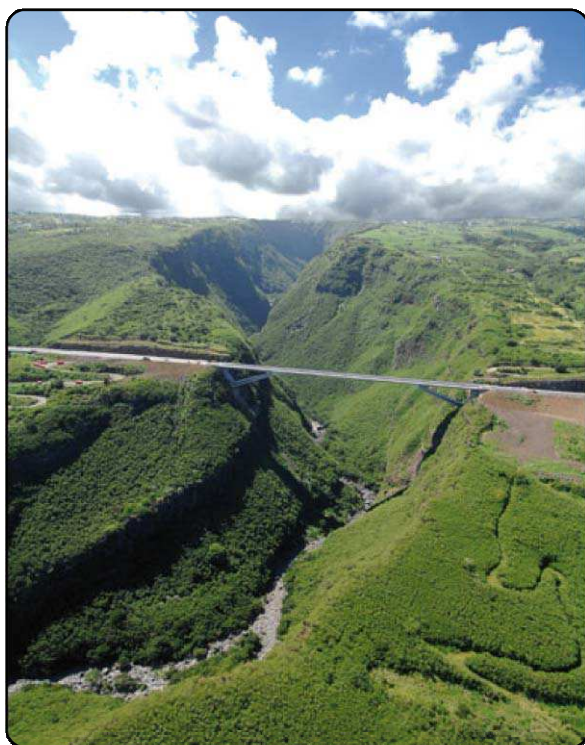
Figure 87: Viaduc de la Grande Ravine, Source: www.dodincampenonbernard.fr
