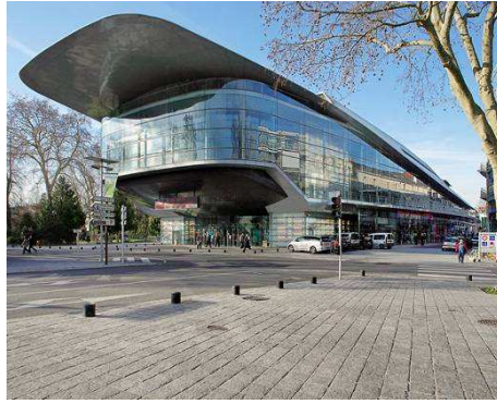
Figure 5 - Photo du Centre Vinci, Tours.
