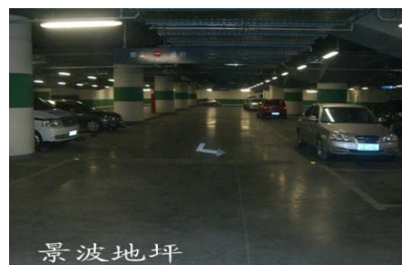
Un parking souterrain
