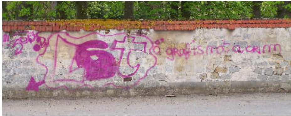
Photo 1: Le mur longeant la sente 14
