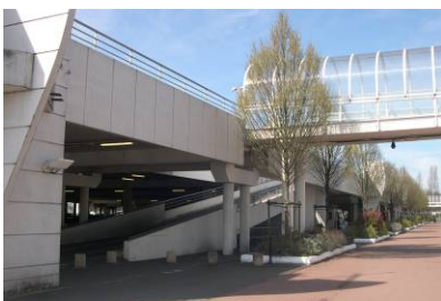
Photo 25: Parking sur dalle
