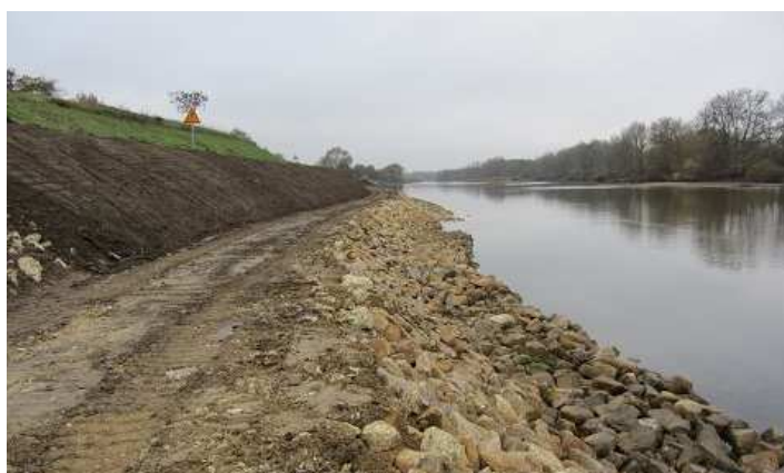
Figure 15: Renforcement pied de digue, Saint Pierre-des-Corps
