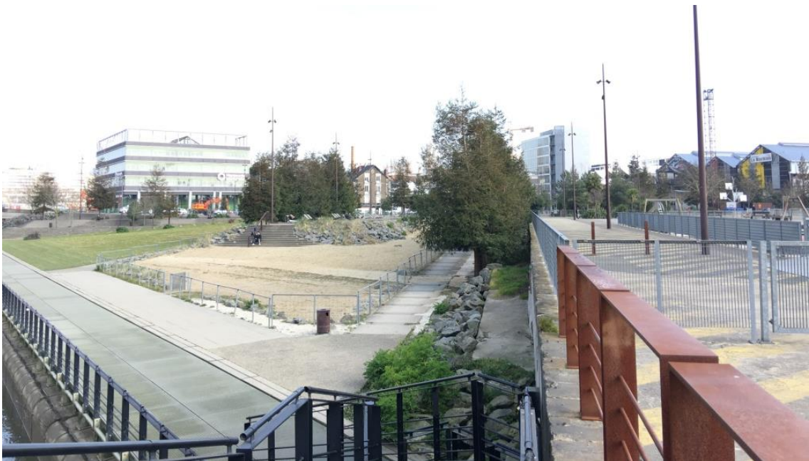
Figure 44. Parc des Chantier (in the beginning of march) Source: Author
