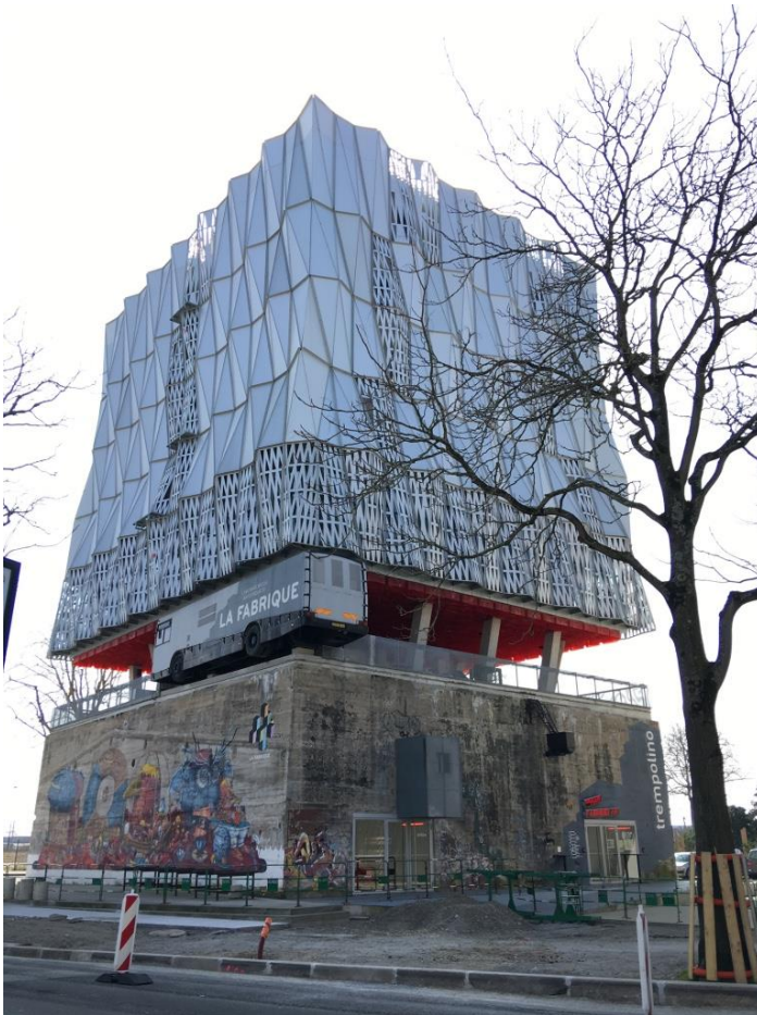
Figure 27. Trempolino Building in the Creative District Source: Author
