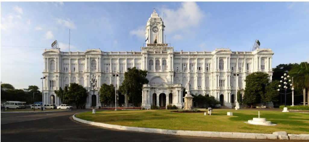
Figure 9: The Rippon Building, seat of Chennai Corporation Sources: http://upload.wikimedia.org/ and personal
